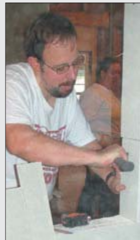
Chris Wood of First UMC in Port Jefferson trims a piece of wallboard.
