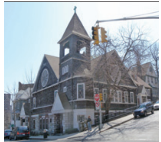
St. Stephen’s UMC in the Bronx will get some exterior restoration.
